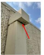
Figure 6 AT.6 - Rusting bearing plates
