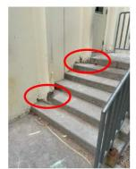
Figure 3 AT.3 - Freeze thaw damage in wall webs
