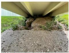
Figure 5 AT.5 - Erosion at bridge connector
