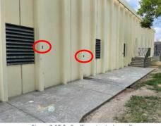
Figure 2 AT.2 - Spalling at exterior wall
