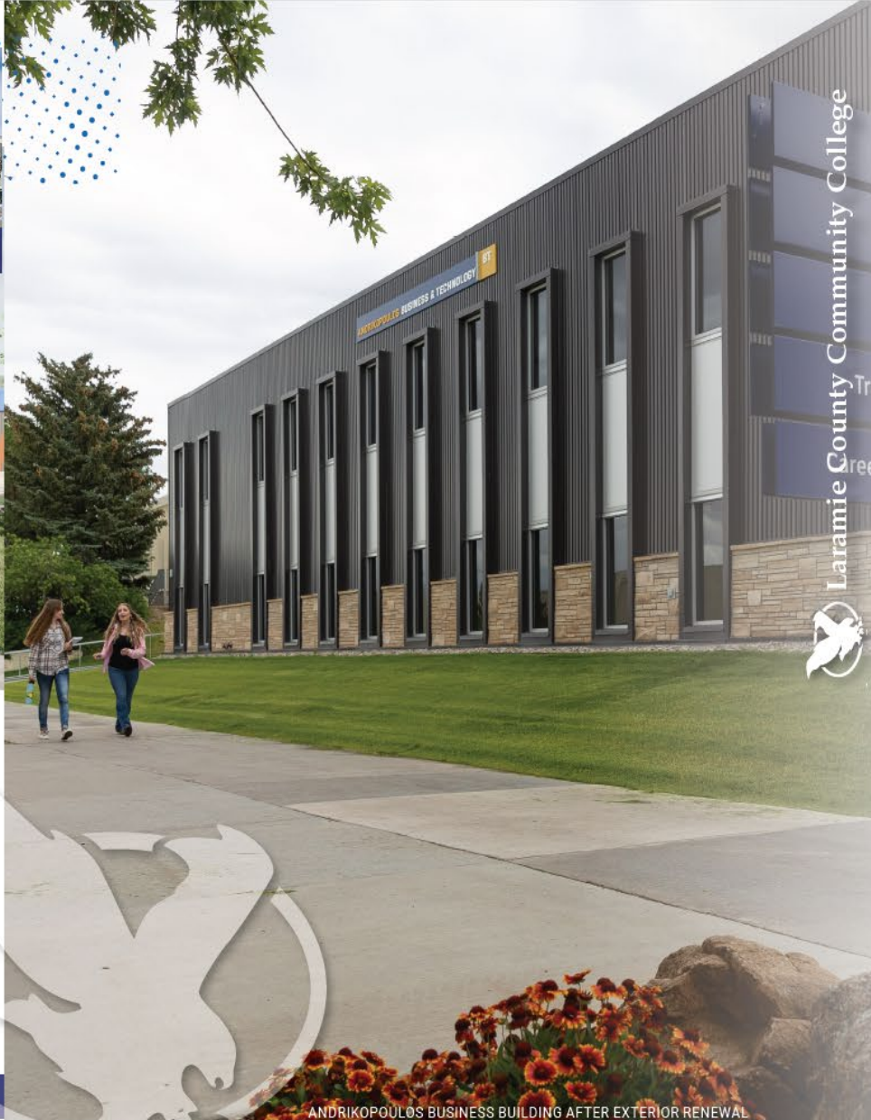
ANDRIKOPOULOS BUSINESS BUILDING AFTER EXTERIOR RENEWAL
